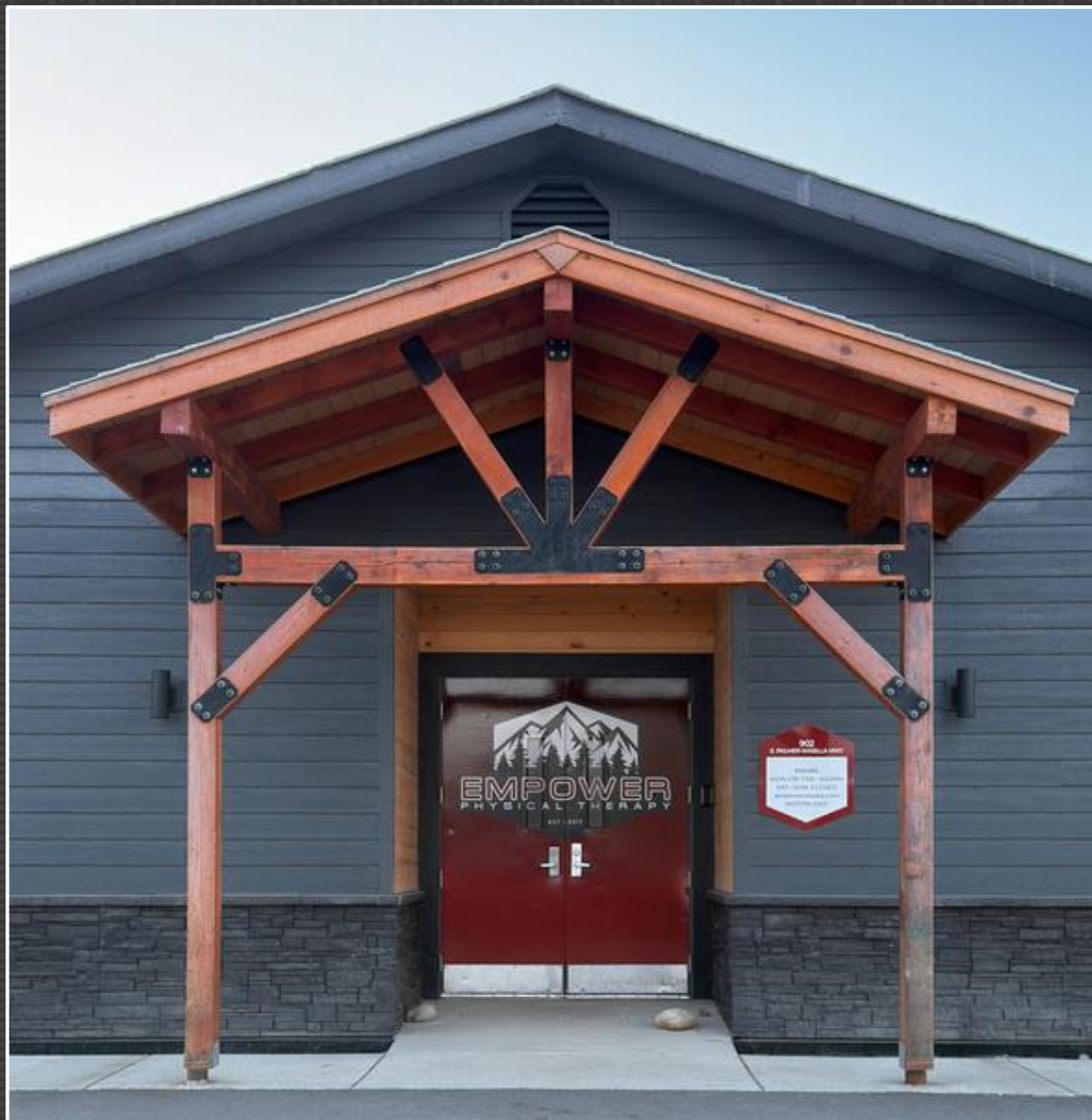
851 a-Chuck Iliff – Grateful - Healthy Repairs
