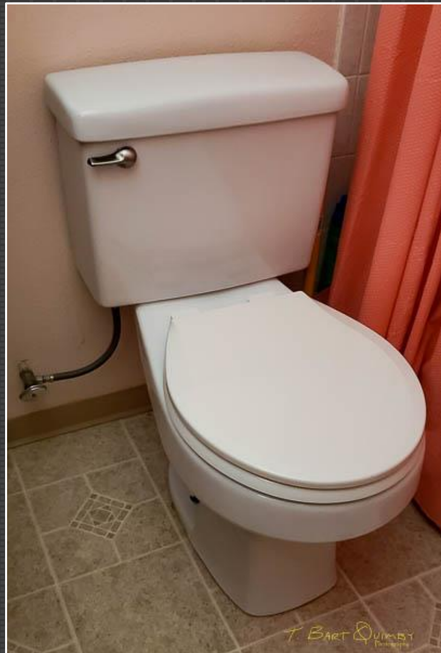
810b-Bart Quimby – Plumbing
