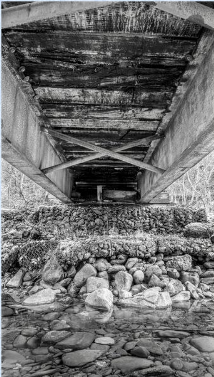
712b-Doug Poage – Bird bridge gabion and girder
