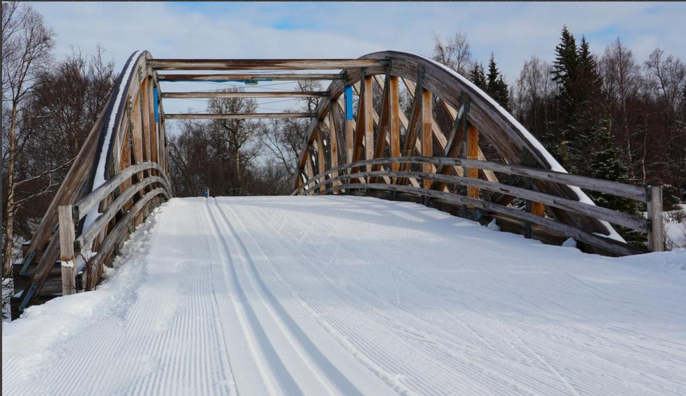
804-ADW – Kincaid Ski Bridge
