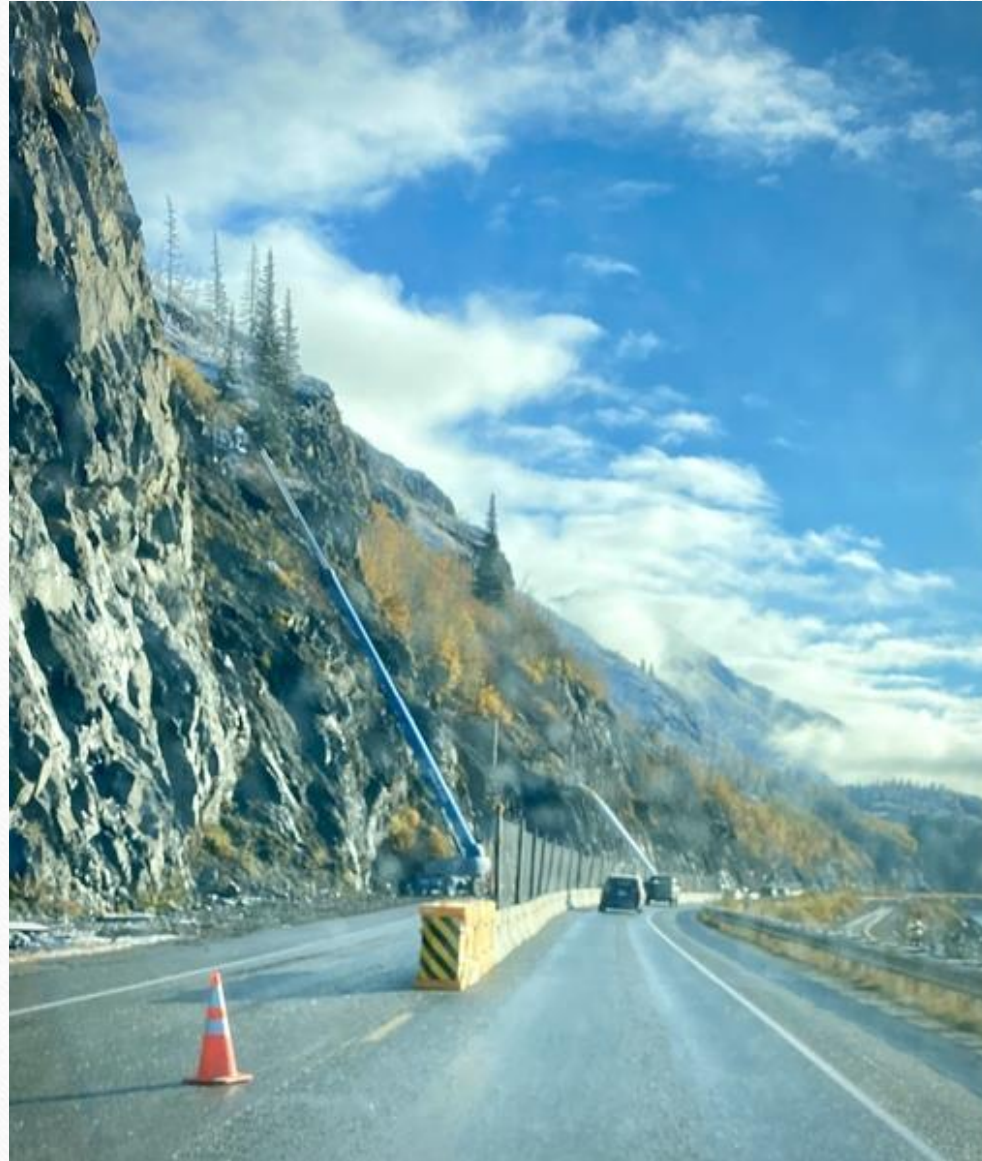
14 - Shirley Mathews - Road Construction
